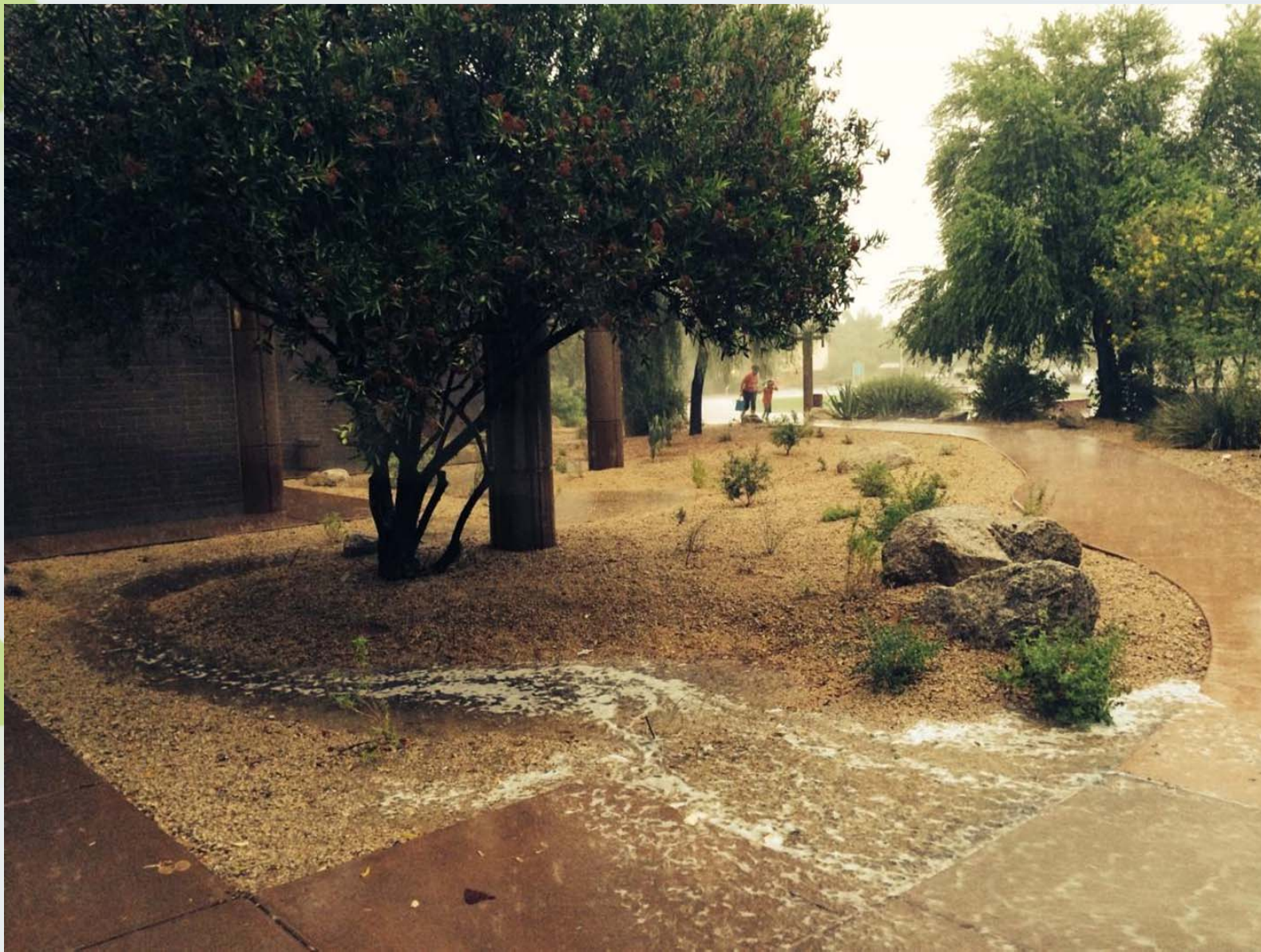
Rain Garden at Glendale's Main Library
