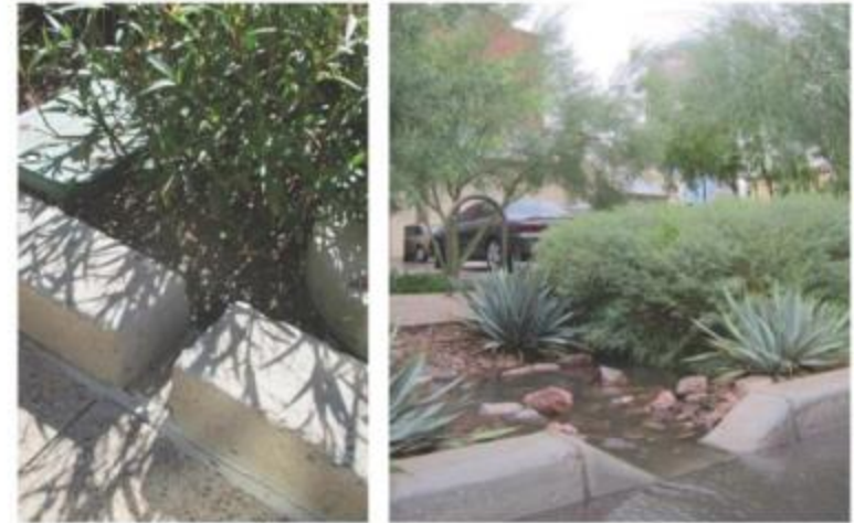
Curb cuts control stormwater flow from streets to LID facilities.
