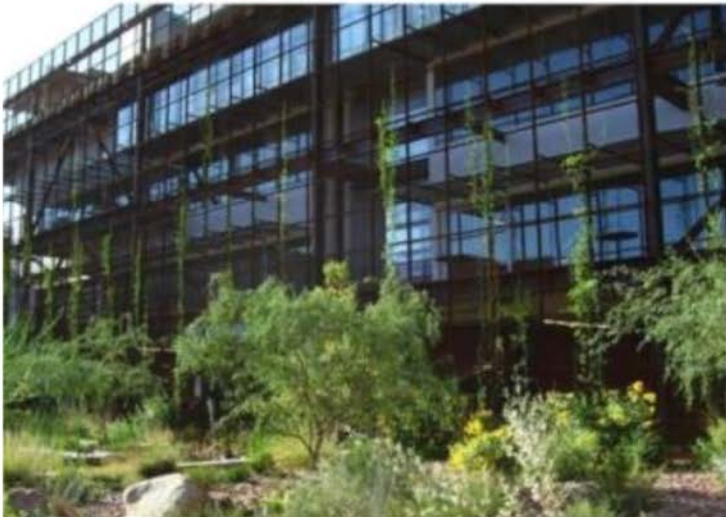
New entry and garden/outdoor classroom provide cleansing garden for adjacent building and pavement runoff.
