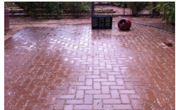
Permeable paver patio Courtesy Summer Waters, UA Cooperative Extension
