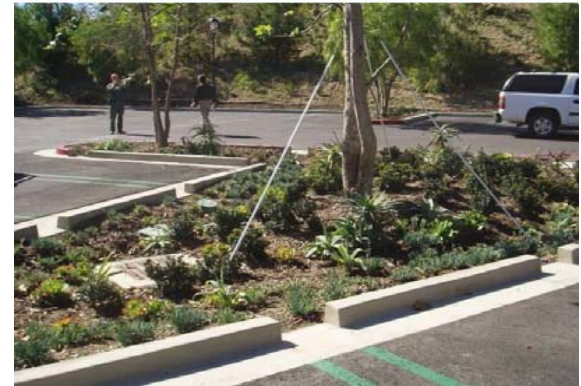
Parking lot runoff captured by bioretention in parking islands Courtesy City of Phoenix
